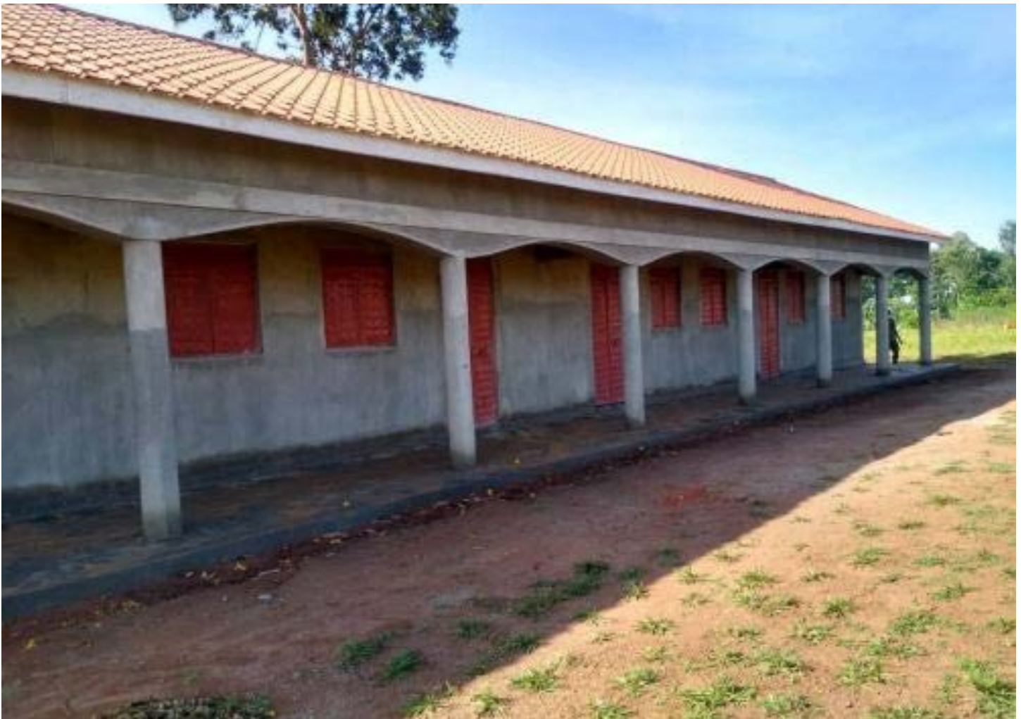
Early Childhood Education Center, Kidera, Tororo District, Uganda (Currently under construction)
